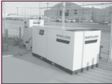
Ingersoll Rand Rotary Air Compressor, Mdl. SSR-EP100, 446 CFM, 100 HP Ingersoll Rand Air Line Dryer Mdl. DXR-600, Built in 1999
