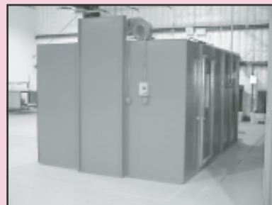
Spray Systems Inc. Small Paint Booth (Paint Storage Room), 15' D x 10'6" W x 8' T w/Explosive Proof Lighting and Sprinkler System, Water Filter System Red Devil Speed Demon Paint Shaker Several 55 Gal. Barrels of Plastic Media Type V Acrylic Blasting Beads
