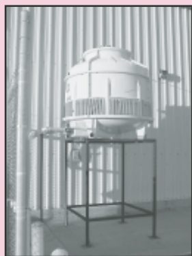
RSD Mdl. 130 Cooling Tower
