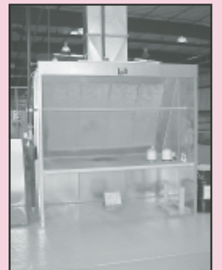
(3) Spray Systems Inc. Paint Booths w/ Explosion Proof Lights and Sprinklers, 8'4" W x 8' T x 4'7" D
