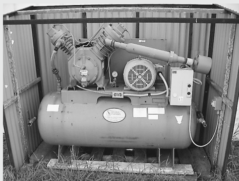
Ingersoll Rand Mdl 71T-2 Horizontal Air Compressor, Dual Stage, 15 HP, 60 Gallon Tank
