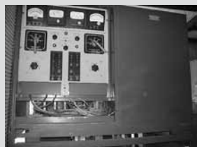
Sun Electric Type A-1 Load Bank, Rating 60 KW, 40 KVAR, 400 Cycles, AC Avionics Instruments Static Inverter Test Bench for Testing Mdl 1A700 (1A) & 1A700 (1B) & (1C) Inverters
