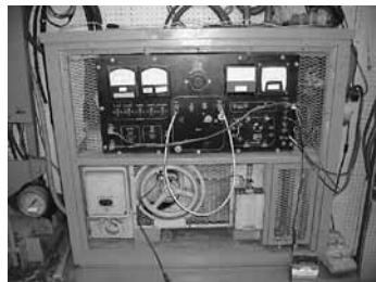
US Vari-Drive Starter Generator Test Bench, Dual Head 2,350-9,000 RPM Low Side, 3,000-11,600 RPM High Side, 600-Amp Load Bank w/Blower, 50 HP
