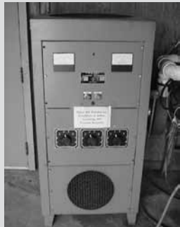
Clinton Mdl S524S0S DC Power Supply, AC Input 230 Volt, 35 Amps; DC Output 4-24 Volts, 500 Amp, 12 KW
