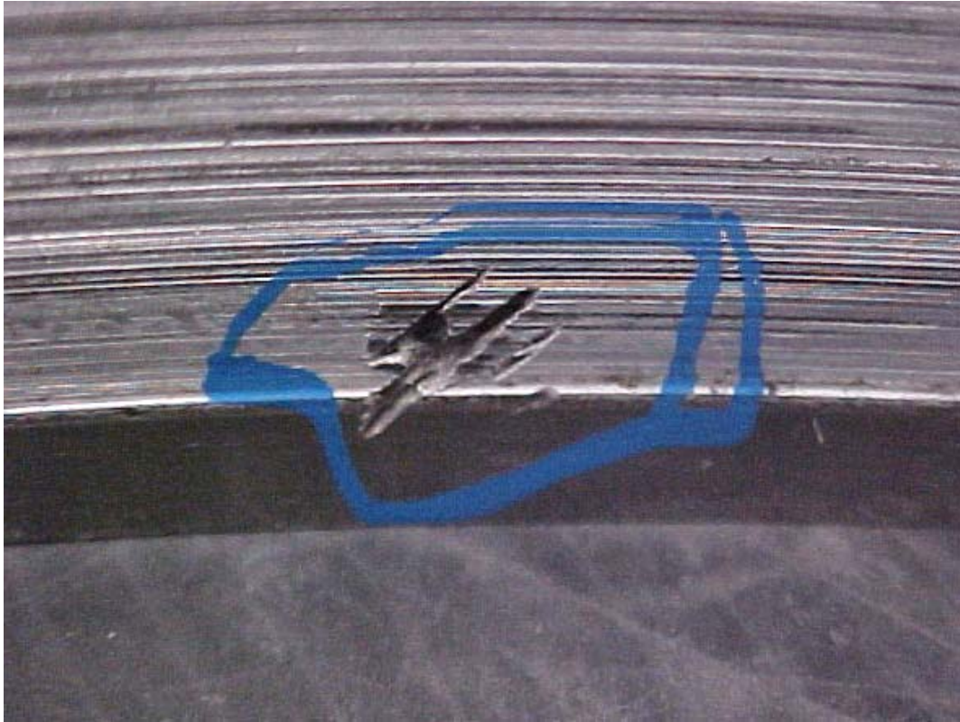
2 ND STAGE LPC STATIONARY SHROUD NICKED ON INNER SURFACE
