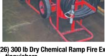
(26) 300 lb Dry Chemical Ramp Fire Extinguishers
