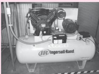
**Ingersoll Rand Mdl 2545 Air Compressor; 175 PSIG, 2 Cyl w/120 Gal Horz Tank**
