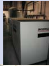
Ingersoll-Rand Mdl SSR-EP100 Rotary Screw Type Air Compressor, Cap 446 CFM Rated Operating Pressure 125 PSIG, 100 HP Motor
