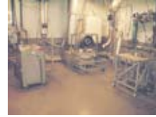
Pneumatic Test Cell #7
